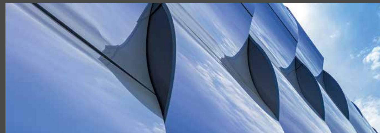
Maxima Shopping Centre, Lithuania | Architect: City projects UAB | Material: ALUCOBOND® PLUS spectra
