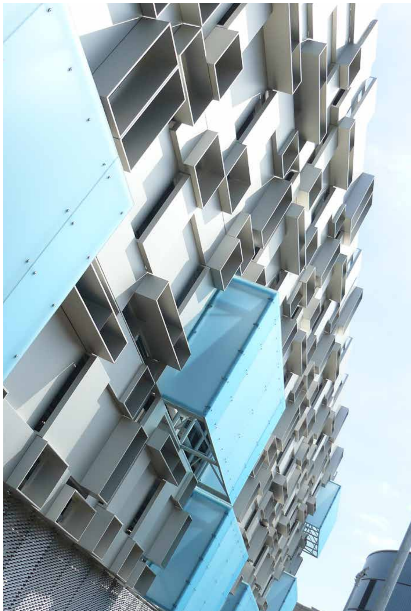
Façade de parking en PERSPEX® Frost Arctic Blue S2 7T77 | ©Photographe: Image Technique
